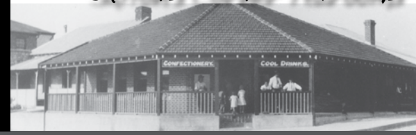
View of Violet Sutton's Corner Tearooms from the Old Mandurah Traffic Bridge
