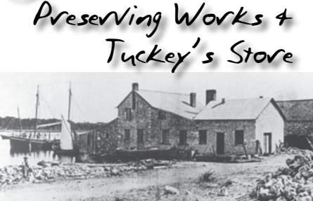
Peel Inlet Preserving Works with storeroom on the right
