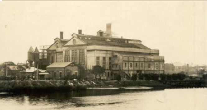
Above East Perth power station circa 1920s. Credit Picture Western Power.
