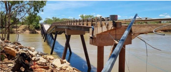
Photographs taken while a relation is working out of Derby with the Main Roads Department. These photographs taken mid—February at a time when the depth of the river was still 6 metres, there is no knowledge of what has happened to the old bridge which remains submerged.
