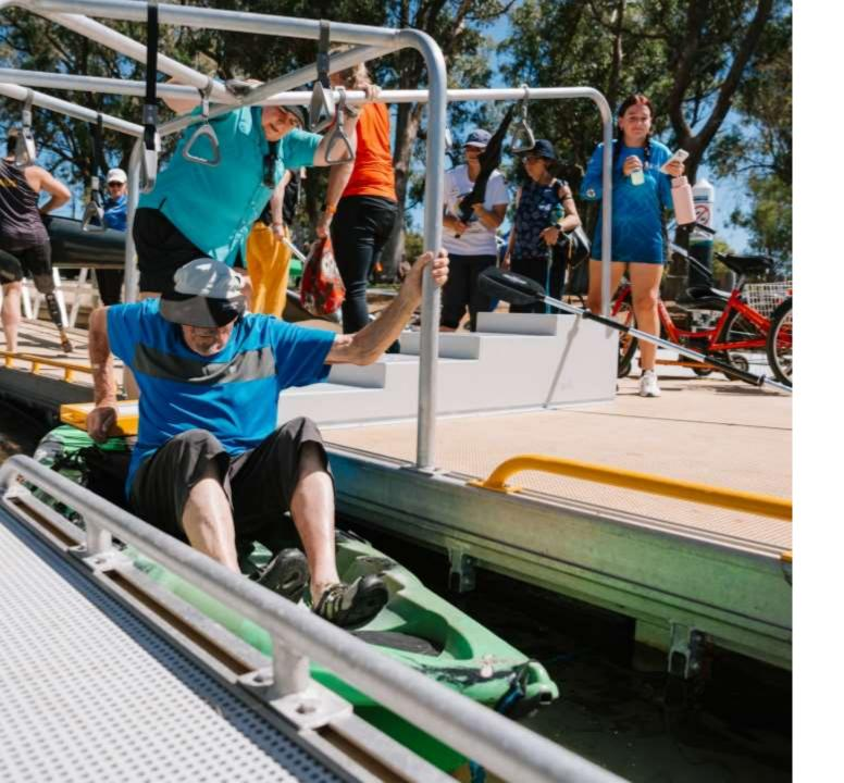
After lowering into the paddle craft, I will retract the bench seat and use the grab rails to push out into the river.
